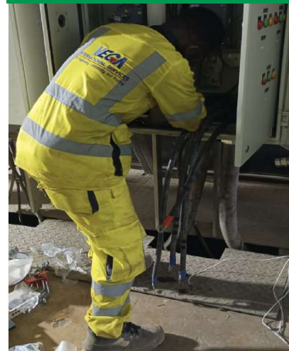
Power Cables Terminations.
