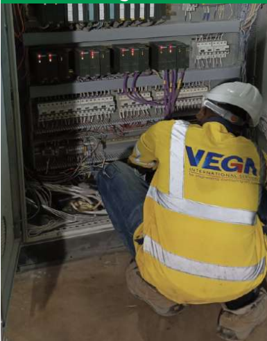
Wiring of I/O Cards and Troubleshooting of Signals.
