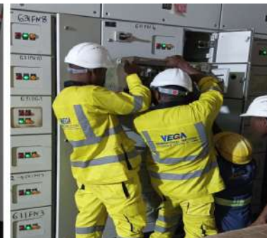
Wiring of I/O Cards and Troubleshooting of Signals.
